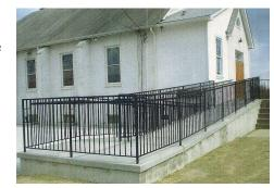
11. <u>34-38" handrails are on both sides of ramp/ stairs, lower railing</u> no higher than 4" above deck, or entrance is level. (S)
